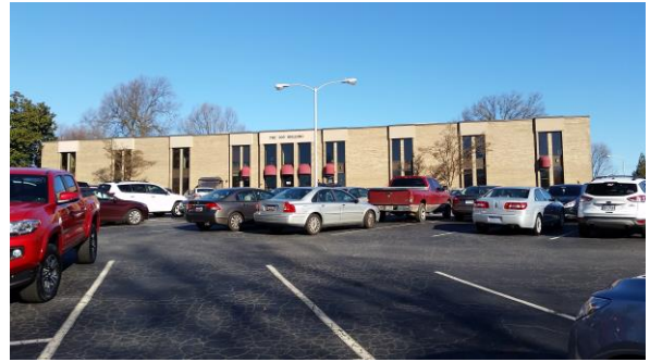
Photo #8 Typical view of site looking north
