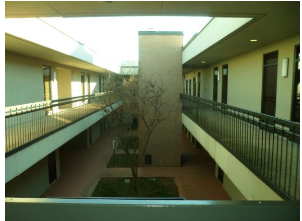
Photo #26 View of open breezeway on second floor looking west
