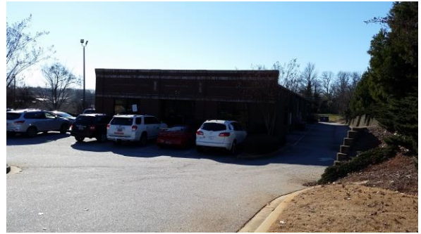
Photo #32 Adjoining property east (Godshall Staffing – 310 University Ridge)
