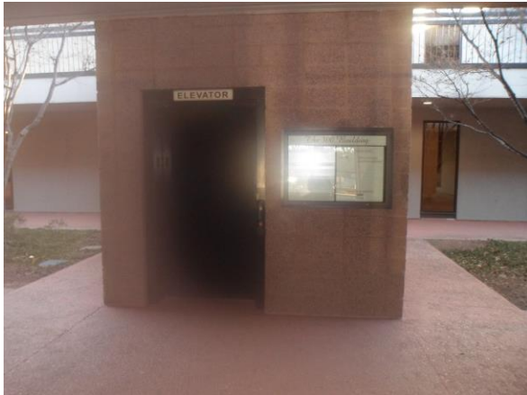
Photo #13 View of elevator centrally located in site building
