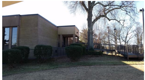
Photo #12 View of western property boundary looking south
